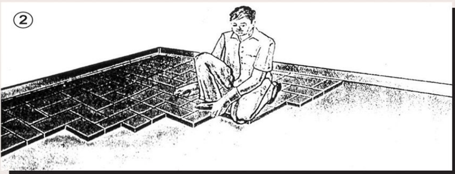
Ensure the Pavers are Layed closely
