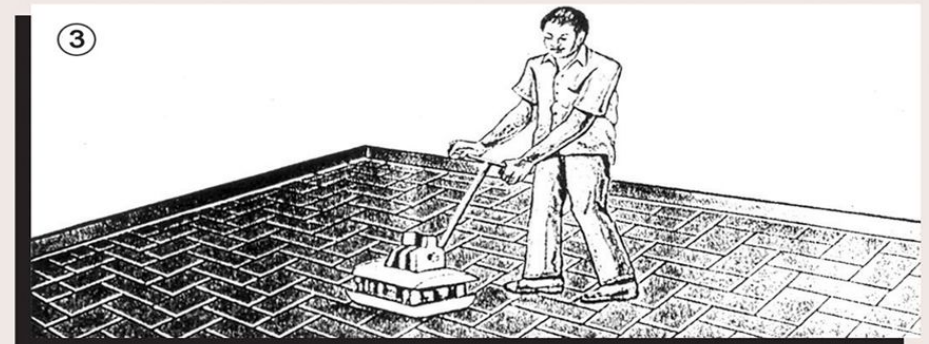
The Pavers are compact for uniform surface
